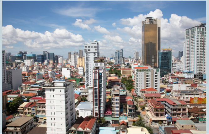
High rise buildings in Phnom Penh
